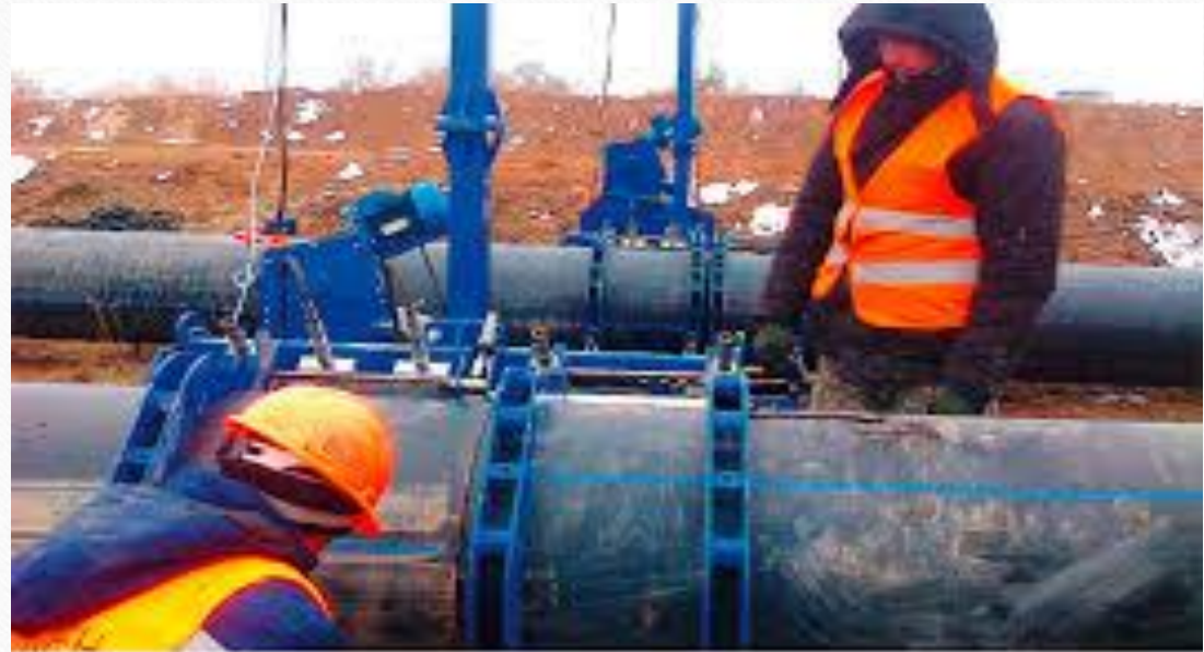
CONSTRUCTION OF WATER MAIN AT THE FEZ "HIMPARK TARAZ"
